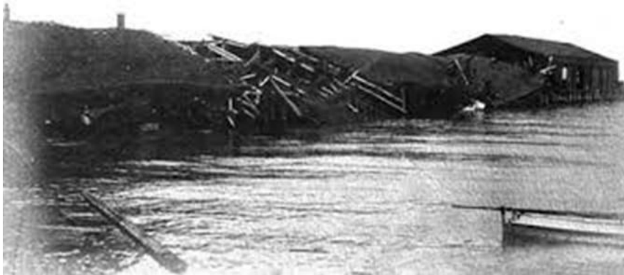
Figure SEQ Figure \* ARABIC 5. Historical photograph of the Pacific Lumber Company dock at Fields Landing that collapsed from liquefaction triggered by the 1906 San Andreas fault earthquake. (Image reproduced from Dengler, 2008, her Figure 8.)
