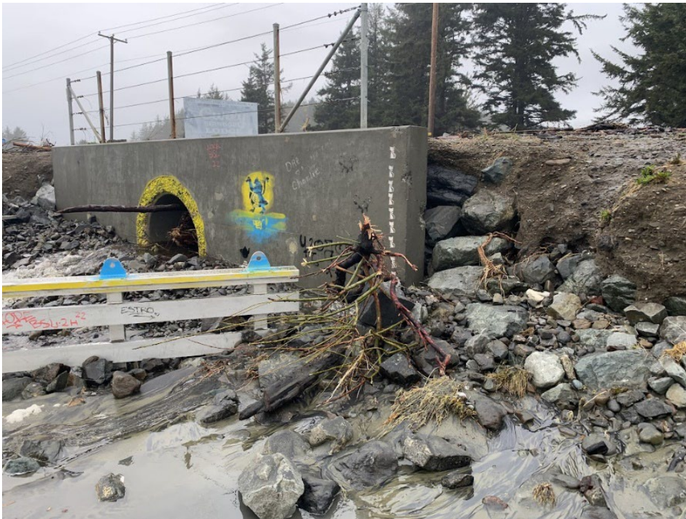
Figure 9. Debris stuck in the culvert entrance and scour around the headwall during the January 5, 2023 storm near PM 24.92 (Photo courtesy of Keven Pratt)
