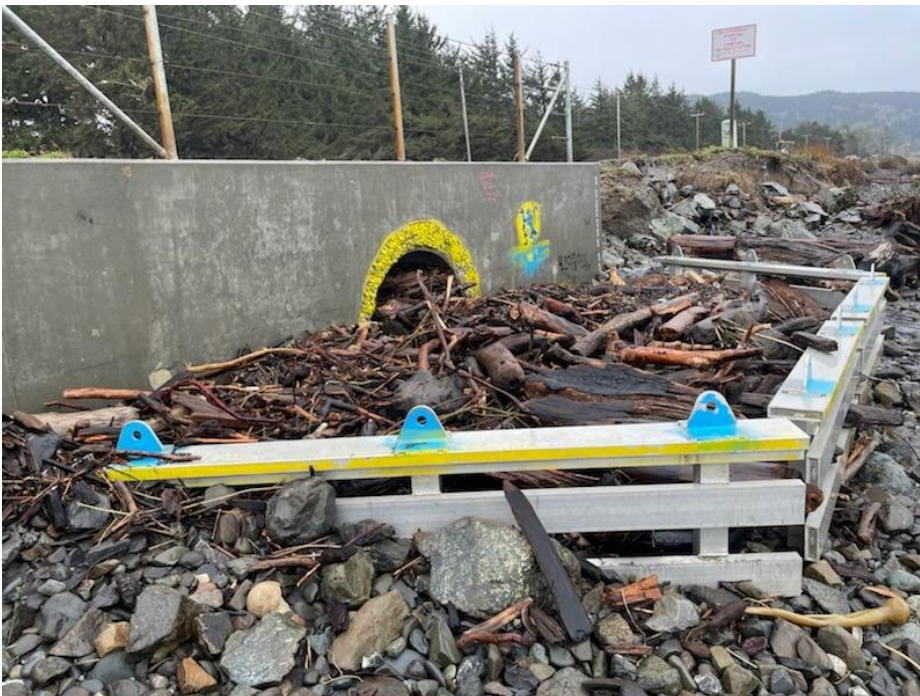
Figure 1-12. Culvert at PM 24.92 filled with driftwood and debris during a January 5, 2023 storm (Photo courtesy of Kevin Pratt)
