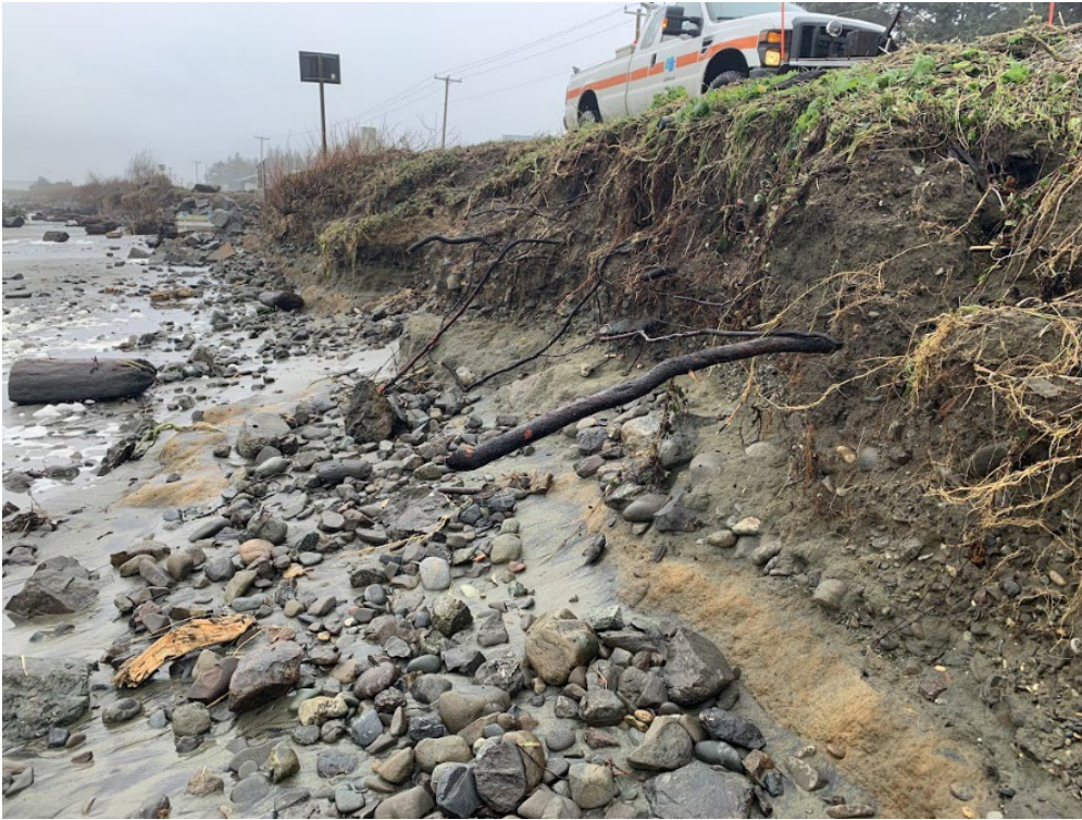
Figure 3-13. Erosion of the berm during the January 5, 2023 storm near PM 24.92 (Photo courtesy of Keven Pratt)
