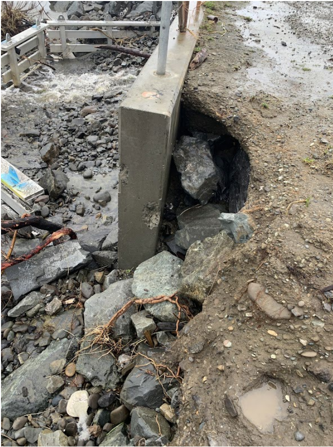
Figure 1-11. Scour at the culvert at PM 24.92 from a January 5, 2023 storm (Photo courtesy of Kevin Pratt)
