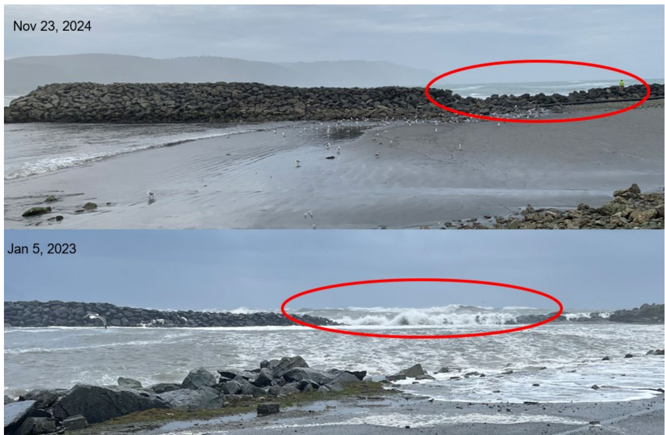
Figure 5-8. Photo showing damaged section of the Whaler Island groin on November 23, 2024 (top) and the damaged section of the Whaler Island groin getting overtopped and flooding of Anchor Way on January 5, 2023 (bottom)
