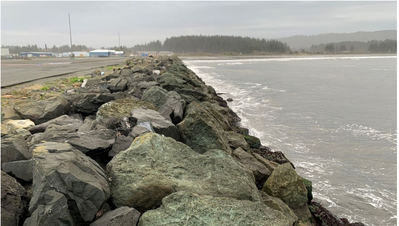
Figure 5-1. Example of a rock revetment (Anchor Way)
