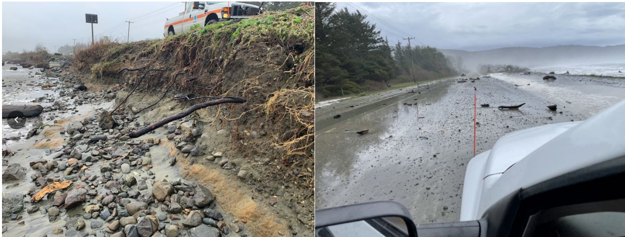
Figure 3-6. Scarping of the berm (left), overwash debris and ponding (right) caused by large waves and elevated water levels on January 5, 2023 (Photos courtesy of Caltrans)
