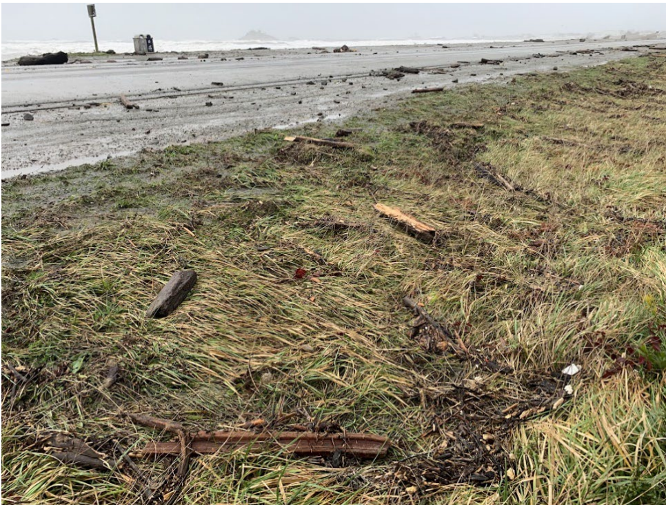
Figure 3-12. Overtopping of Highway 101 during the January 5, 2023 storm near PM 24.92 looking north (Photo courtesy of Keven Pratt)
