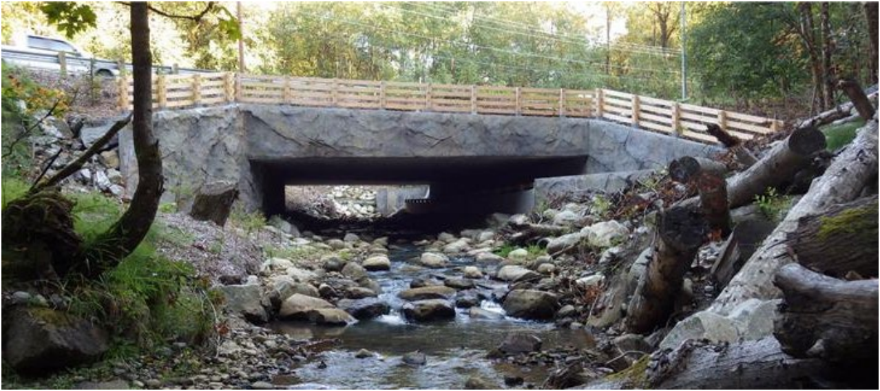
Figure 6-3. Example of bottomless culvert to be used at Culvert 3
