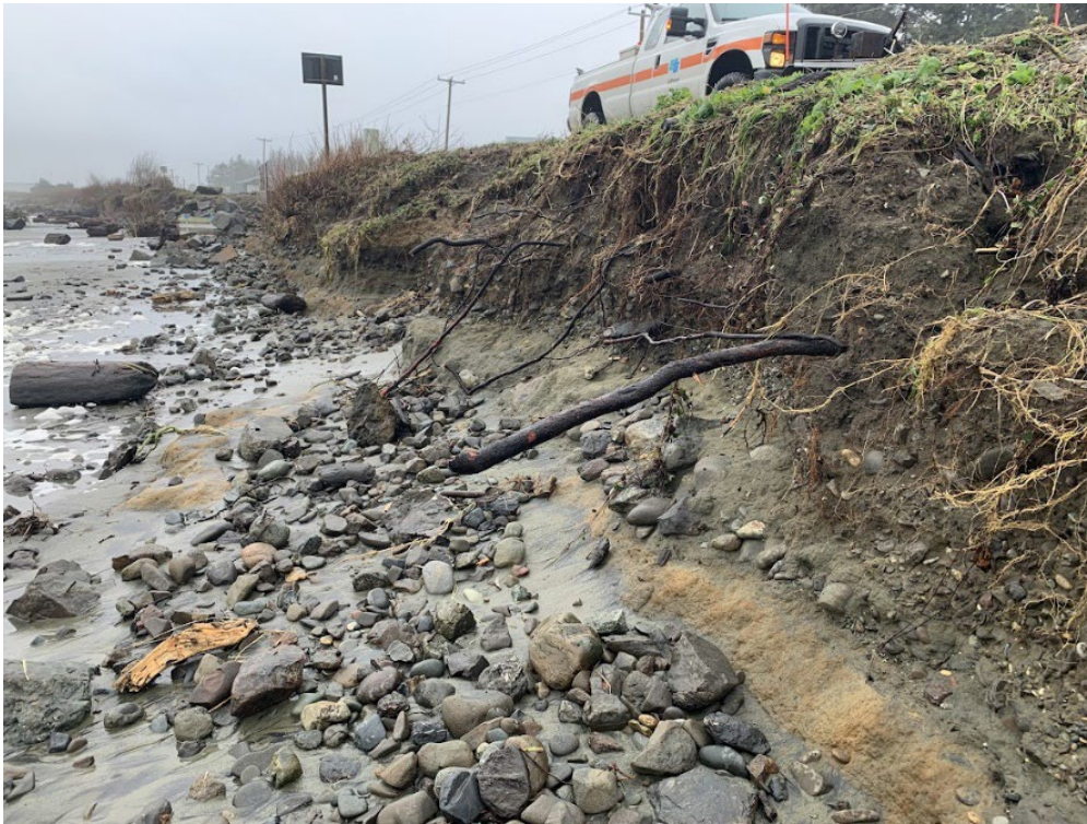
Figure 8. Erosion of the berm during the January 5, 2023 storm near PM 24.92 (Photo courtesy of Keven Pratt)
