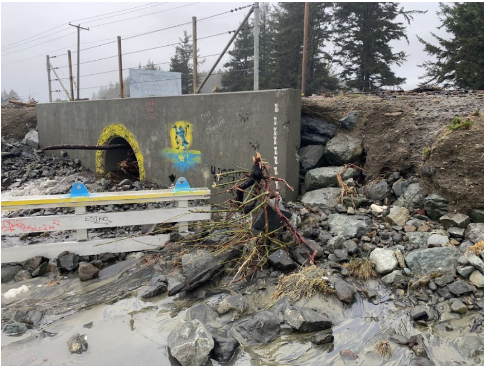
Figure 3-14. Debris stuck in the culvert entrance and scour around the headwall during the January 5, 2023 storm near PM 24.92 (Photo courtesy of Keven Pratt)
