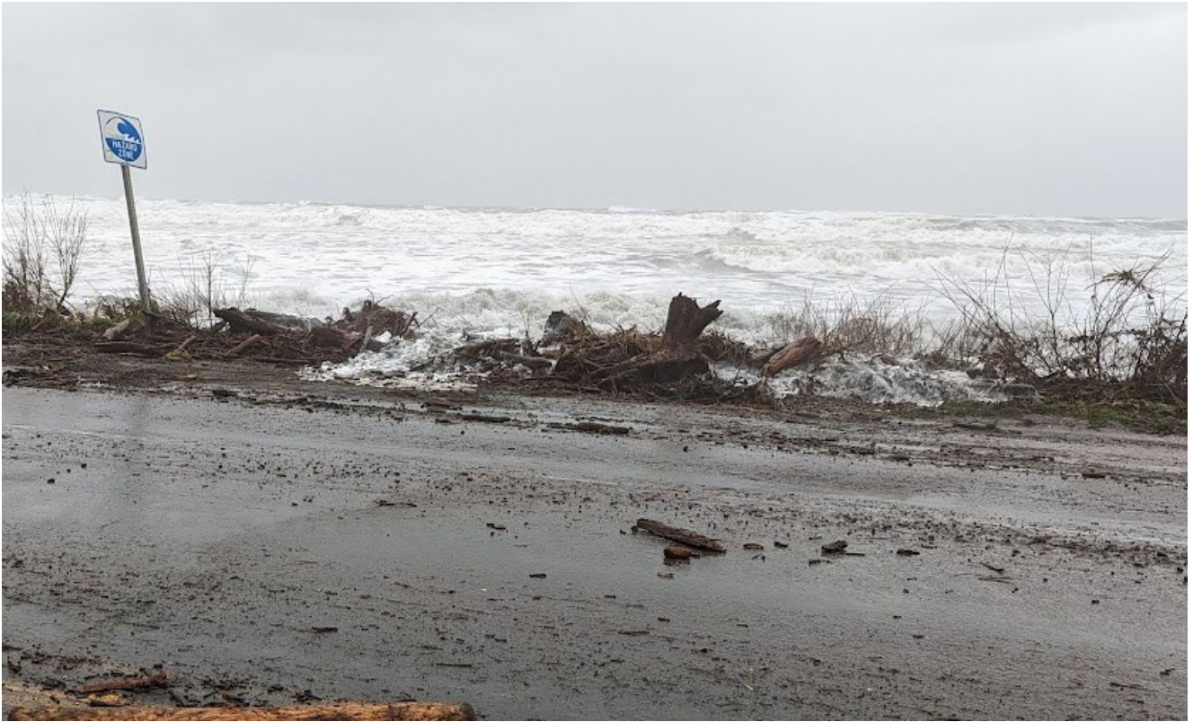
Figure 3-11. Overtopping of Highway 101 during the January 5, 2023 storm near PM 24.92 looking west (Photo courtesy of Keven Pratt)
