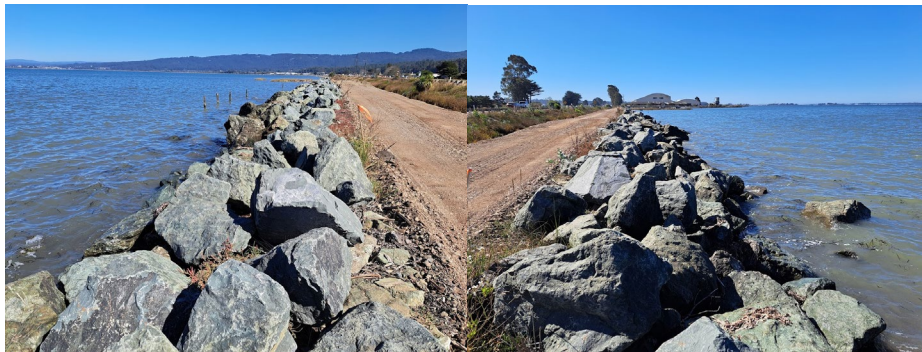
Figure 1.4.5: Extraction Point 4. The location of the actual extraction point is on the mud flat. [Left]: Looking north from the top of the protective shoreline structure which is characterized as Rocky Shore Protection (RSP, or “riprap”). [Right]: Looking south from the top of the protective shoreline structure.
