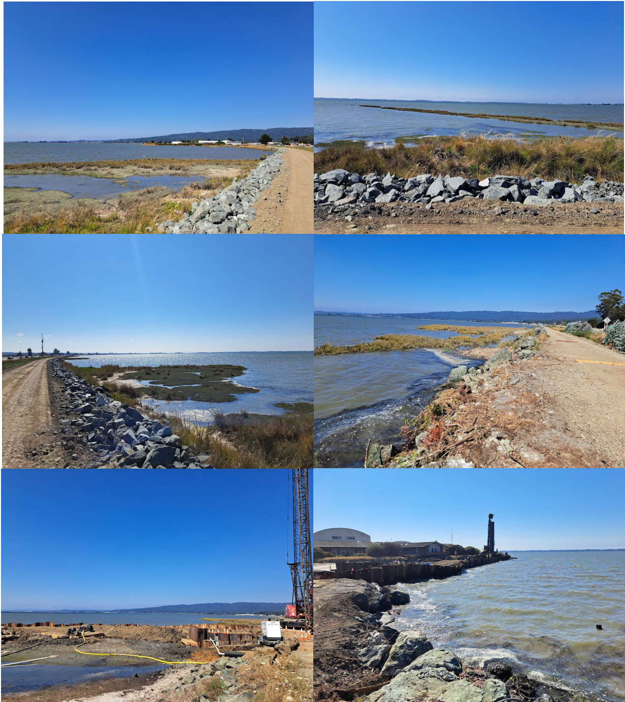
Figure 1.2.2: Photos along Segment B (Figure 1.3) of the corridor shoreline with northernmost photos at the top and southernmost photos at the bottom. This segment is primarily riprap, with a remnant earthen “peninsula” levee (top right, constructed in 1960 as part of an abandoned attempt to expand Bracut; Rohde 2020), and small swaths of salt marsh (center). The bay trail is under construction and abuts the shoreline.
